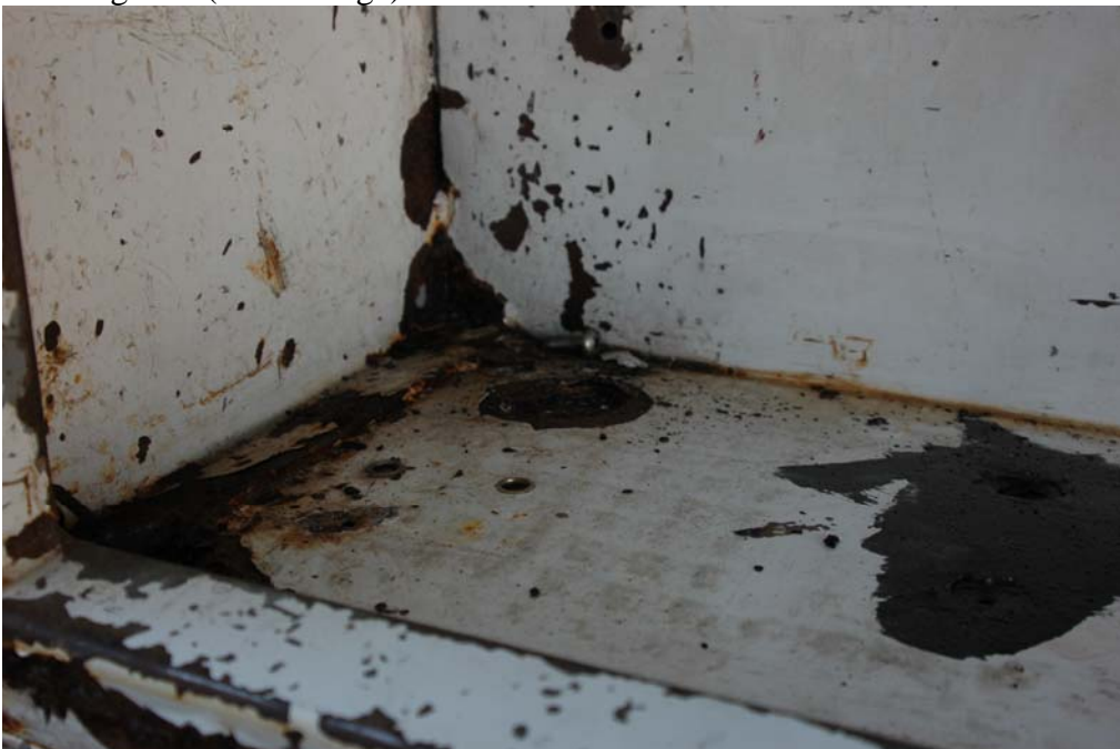
Inside front cabinet damage.
